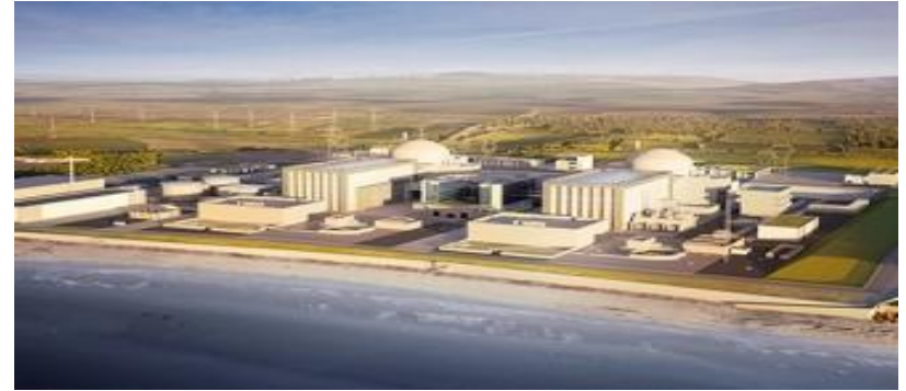
New CFD plant
