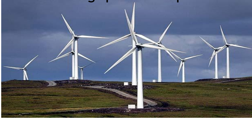
Existing operational plant
