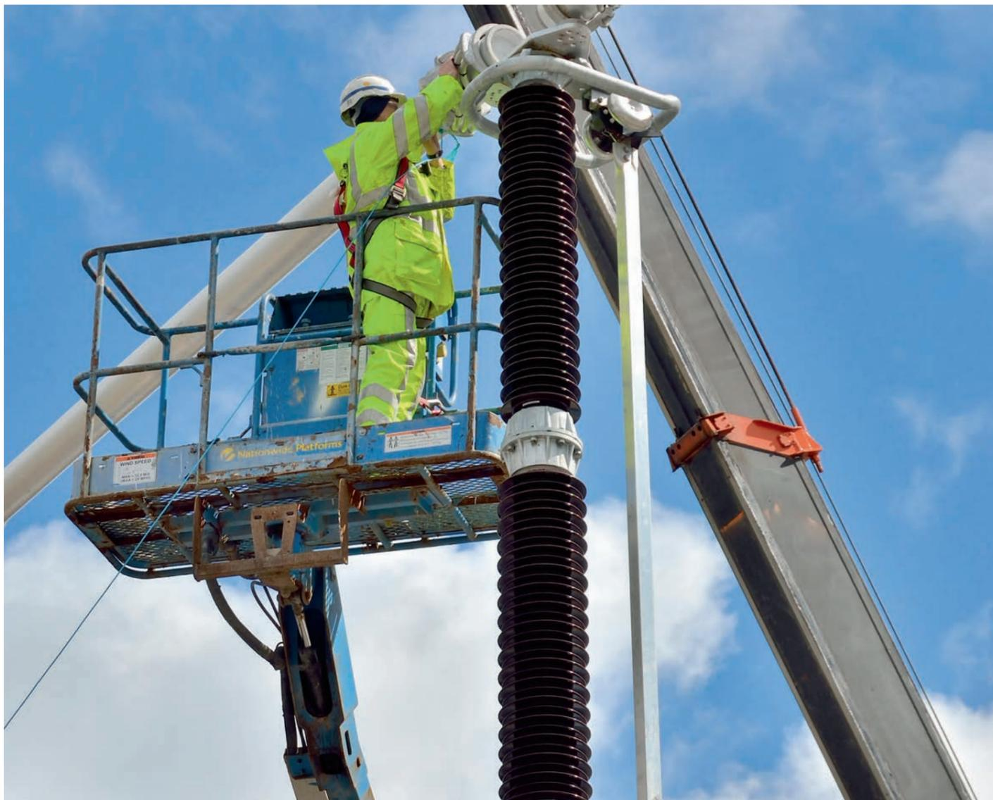
Installing a 400kV Busbar at Moffat Substation
