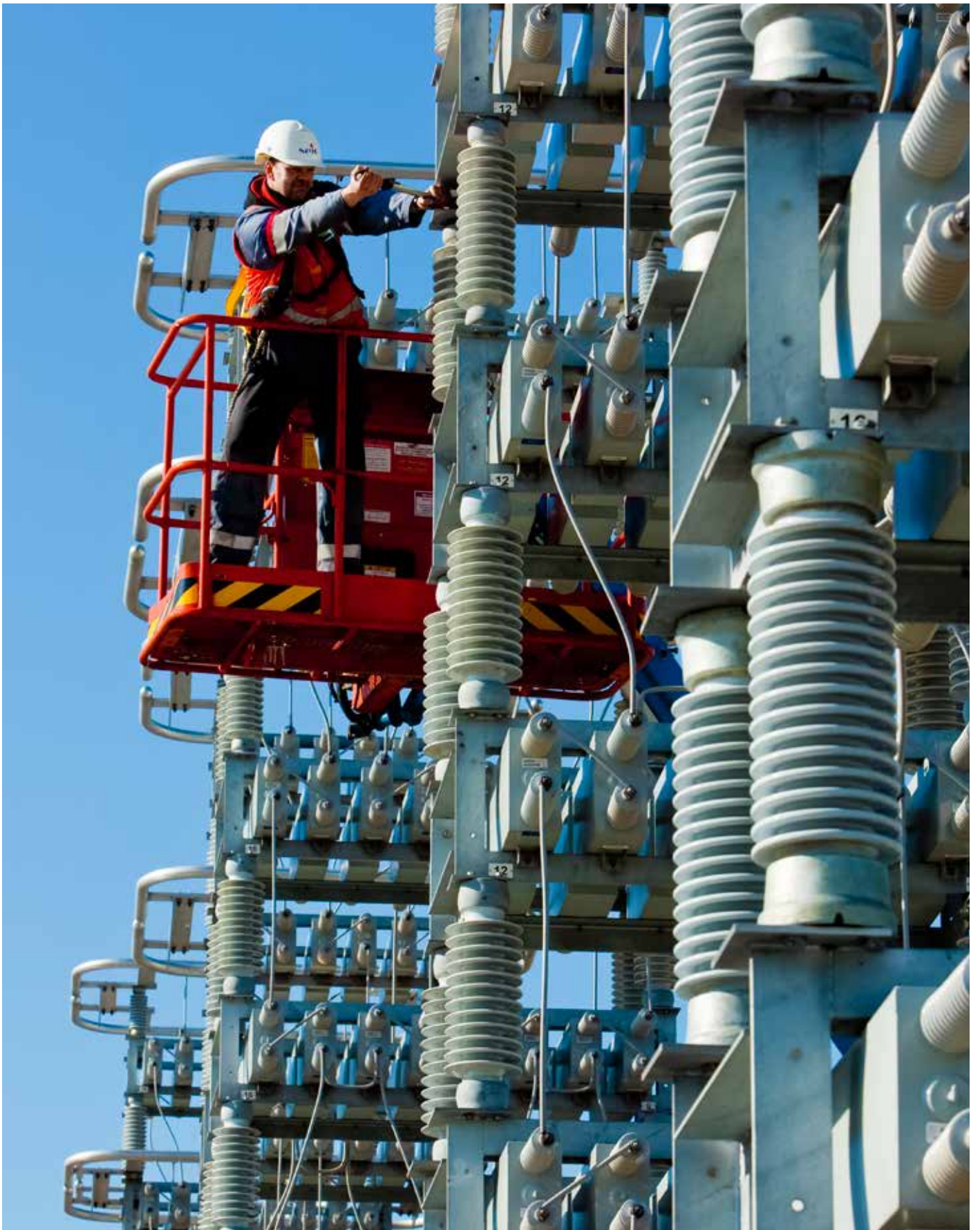
BritNed work in progress
