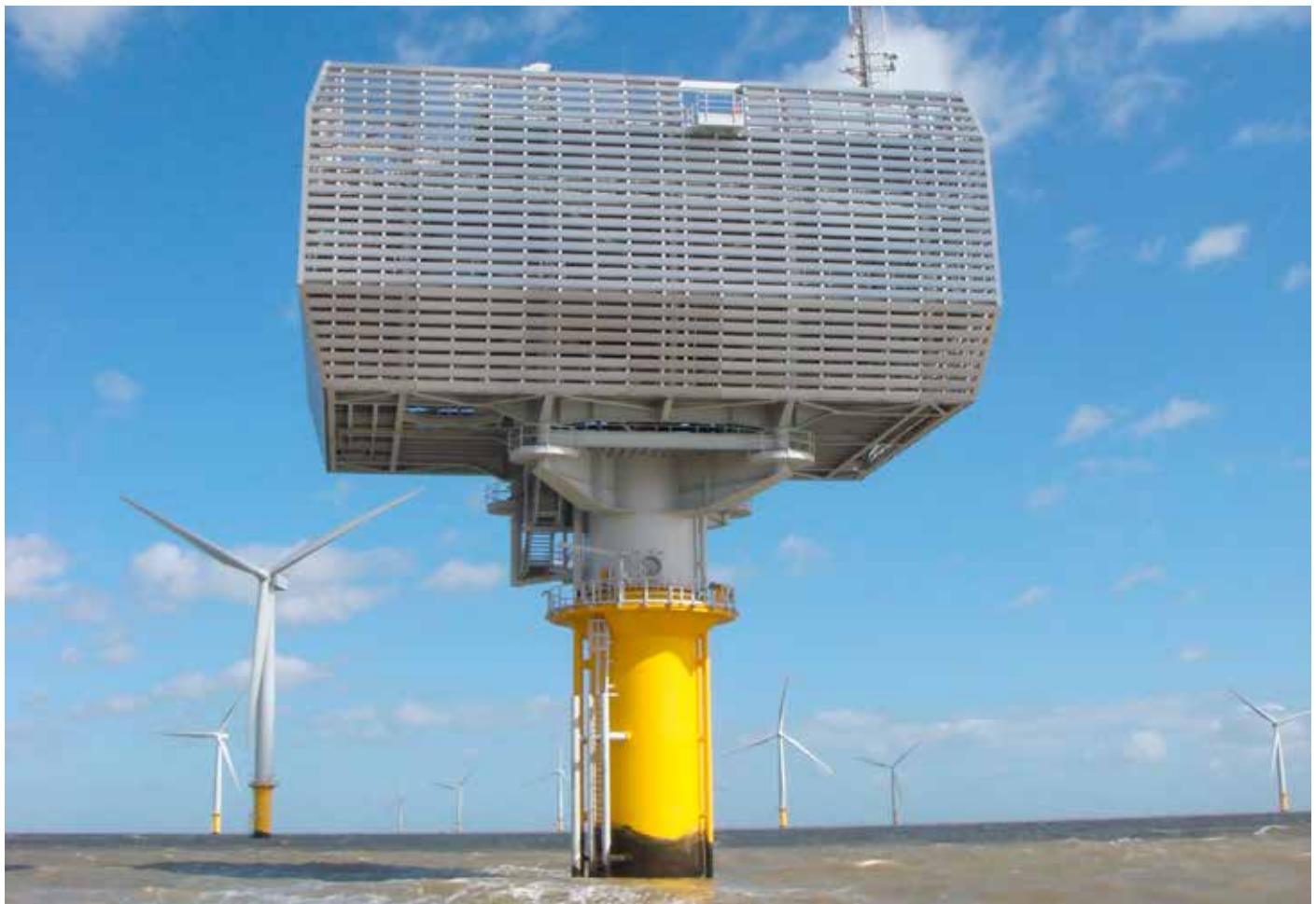
Gunfleet Sands Offshore substation platform
