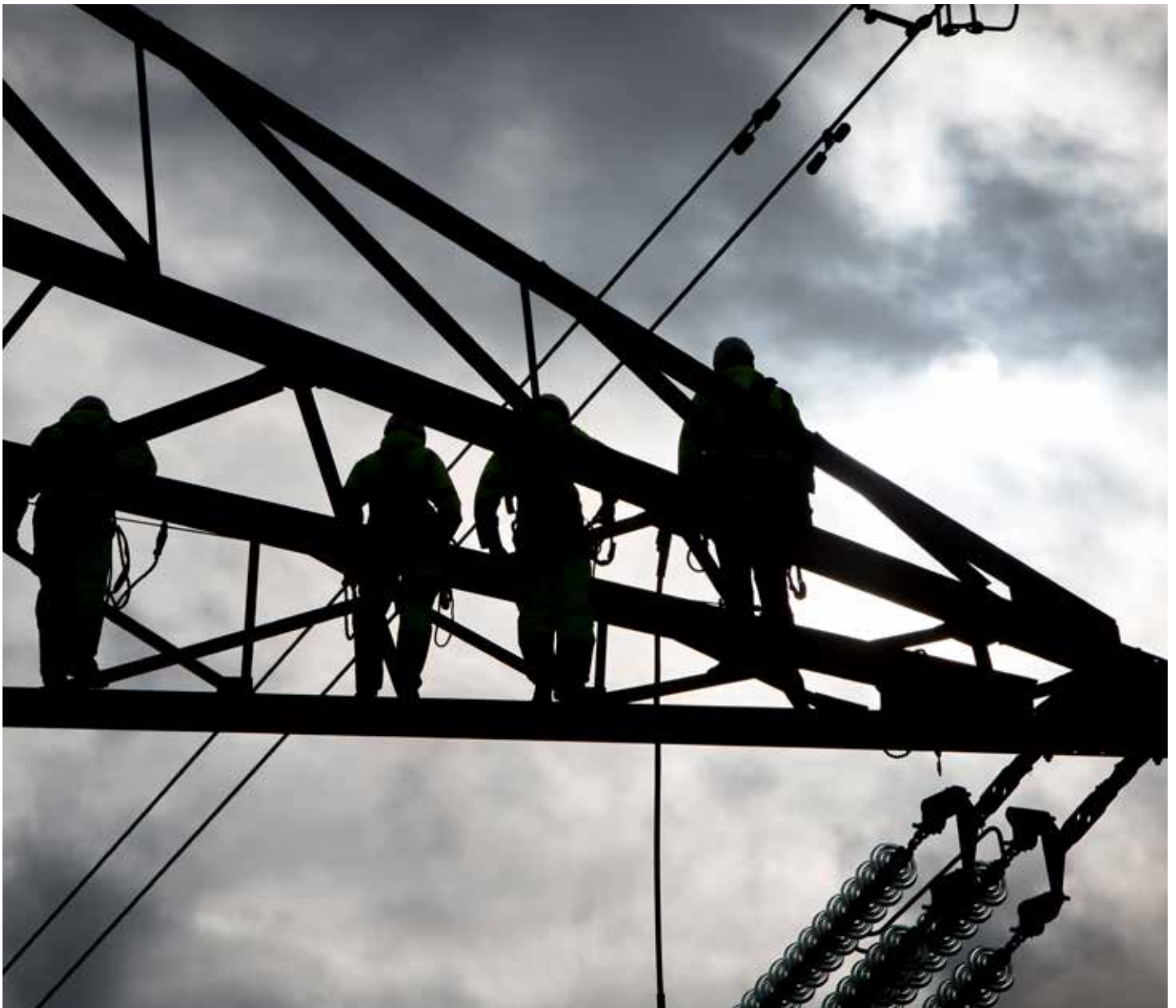
Silhouettes on overhead lines
