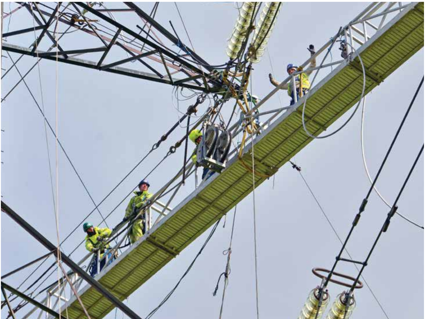
Overhead Line Work at Strathaven
