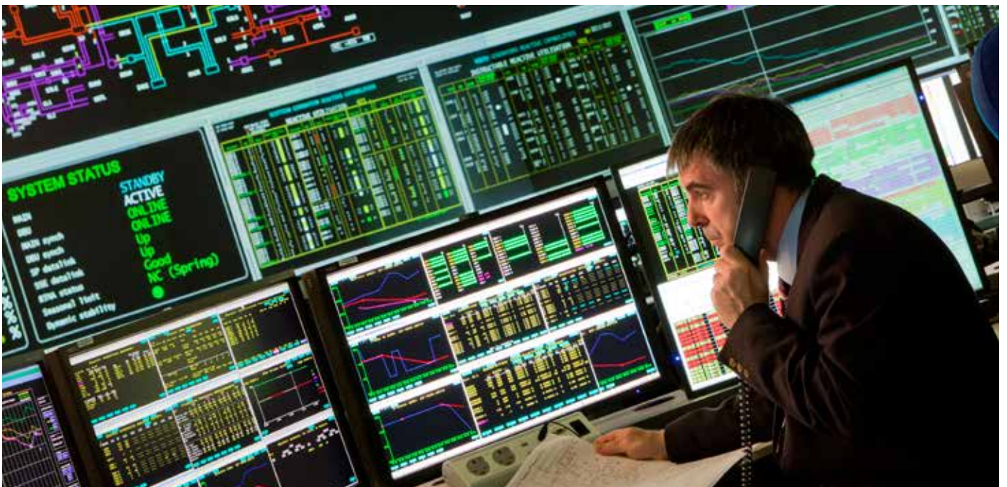
Electricity National Control Centre, UK
