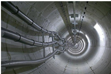
Figure E.8 Transmission cables installed in a 4m tunnel
