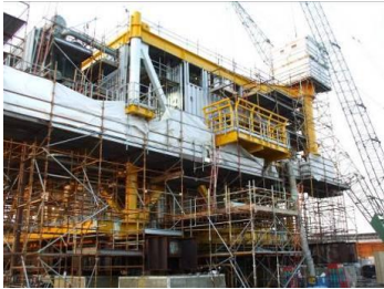
Figure E.15 Thanet substation under construction Image courtesy SLP Engineering
