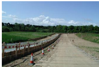
Figure E.13 A typical open trench cable swathe [1]
