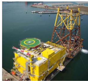
Figure E.16 BorWin Alpha HVDC topsides and jacket. Courtesy of ABB
