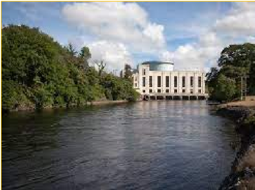
Energised up to 275kV from 13MVA Generator & measure BLPV of Hydro
