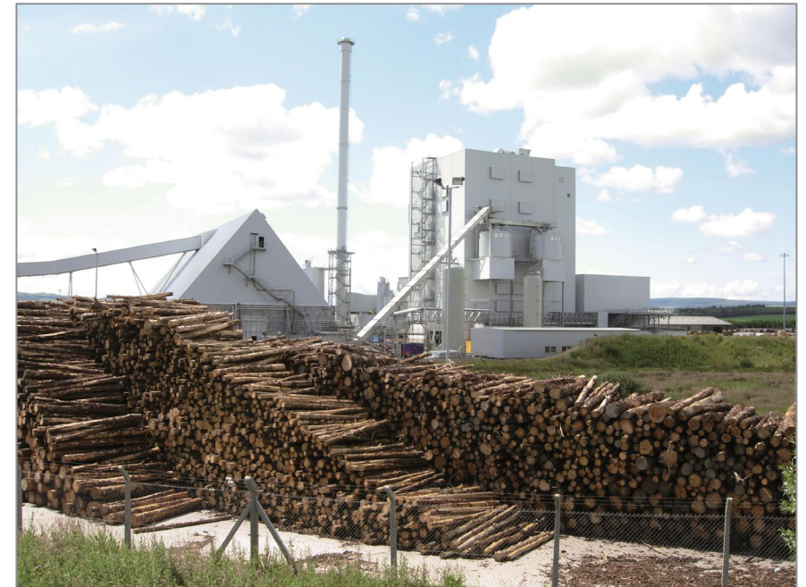
Energised up to 400kV from 53MVA Generator & measure BLPV of Biomass
