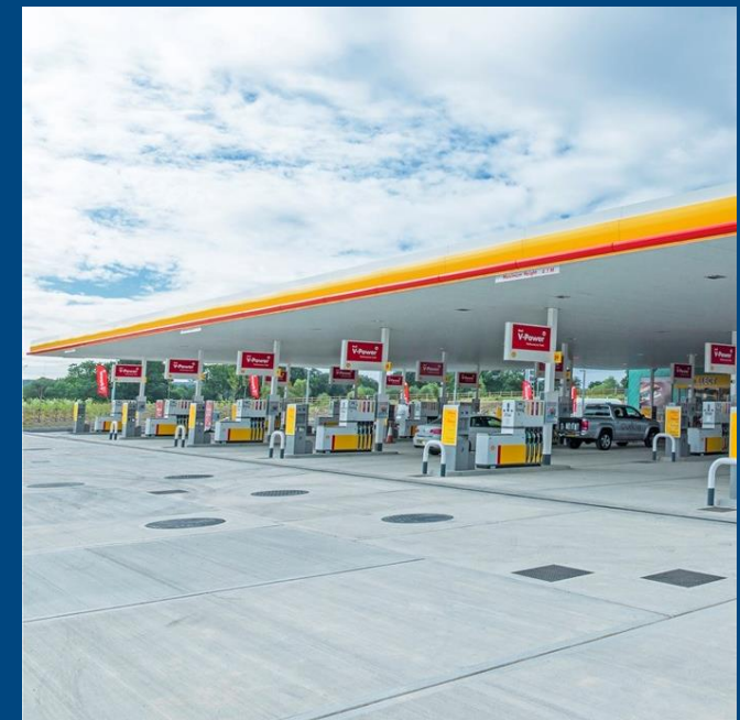
In a charging forecourt
