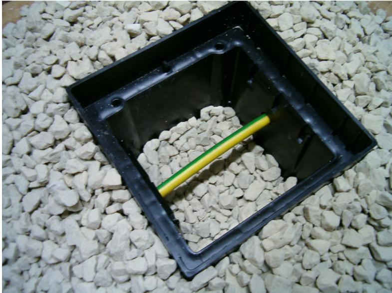
**Figure 1 An example of earthing connection box with test facility\***
