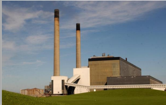
Cockenzie Power station demolition gets under way
